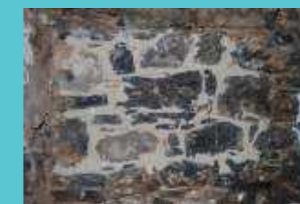
Prefugiranje zidov. Vir: Corradi in sod., 2006
